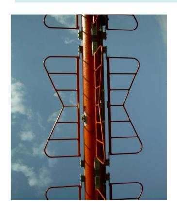
The rectangular area between the inside edge of the element and the support pylon is excited with RF energy, which makes the element radiate. The impedance of the antenna is set by the distance of the support pylon to the inside edge of the element. The typical impedance is 75 to 77 Ohms. The feed harness for the antenna pictured has not been installed yet.
