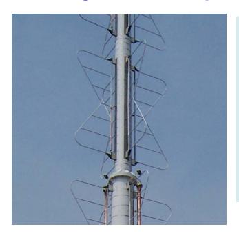
Most high band TV stations use batwing style antennas. It is a design old enough to collect social security. Many of the antennas now in service are over 40 years old. As stations on now on high band look at replacing their current antennas and stations moving to high band, the batwing antenna is worth taking a look at.
